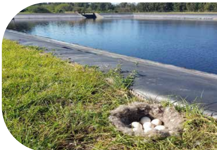
ESUP Dam (Storm Water)
